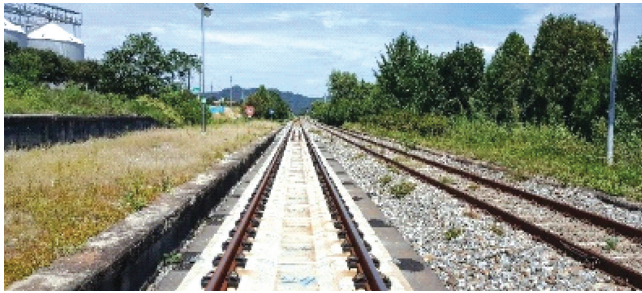
Fig. 3. Asphalt concrete tracks system in Korea
