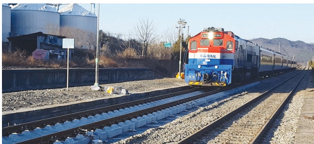
Fig. 4. Trains running on asphalt concrete tracks in Korea
